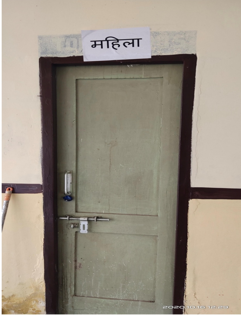
(Disabled friendly washroom)
