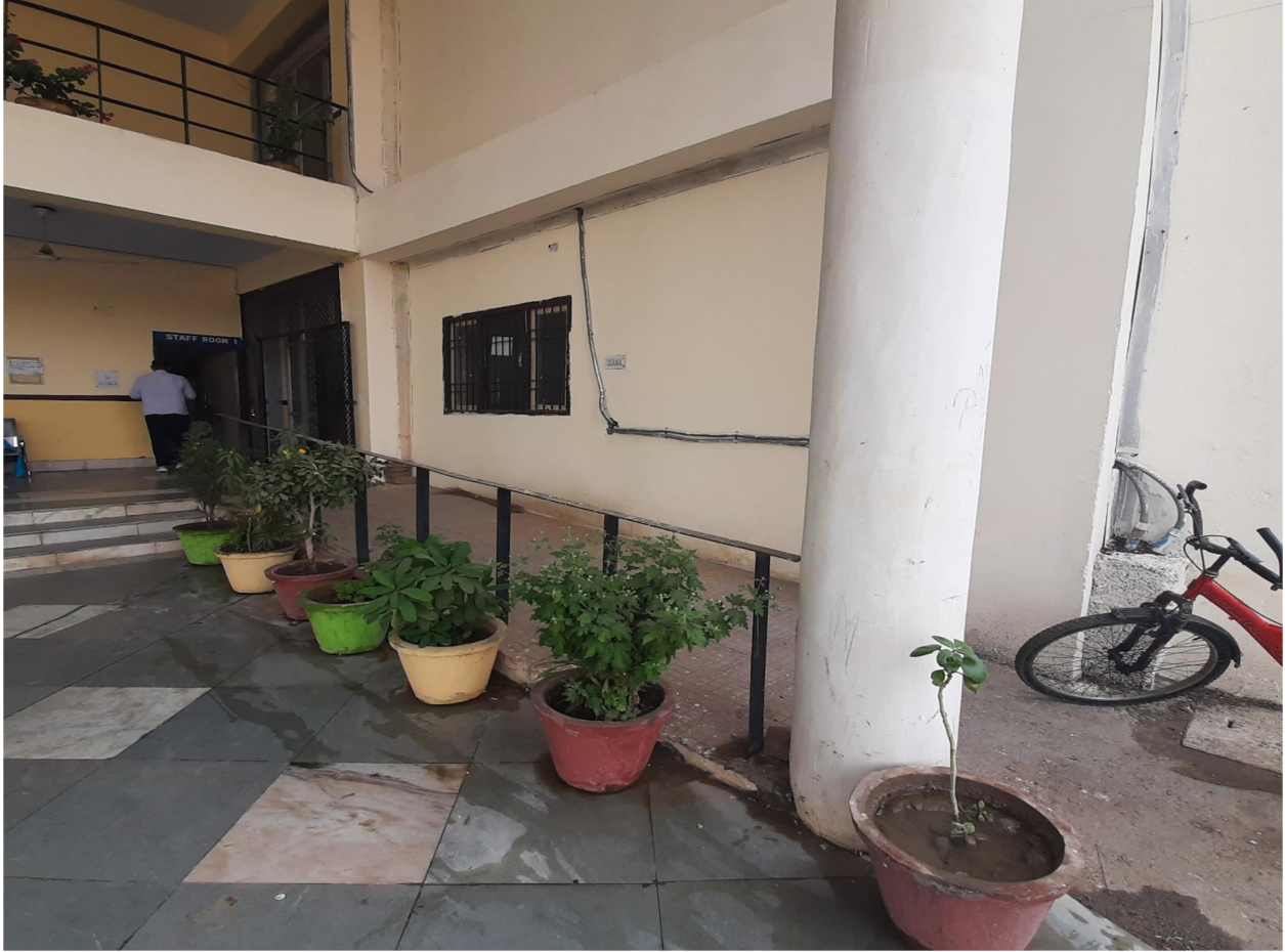
(Ramp for easy access to classrooms)
