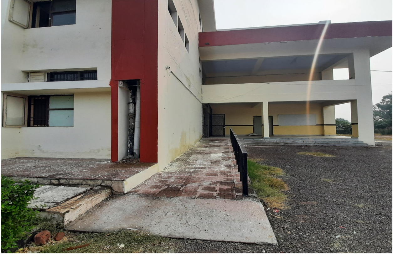
(Ramp for easy access to classrooms)
